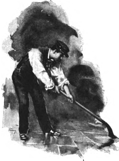
Cutting Open a Tin Roof.
